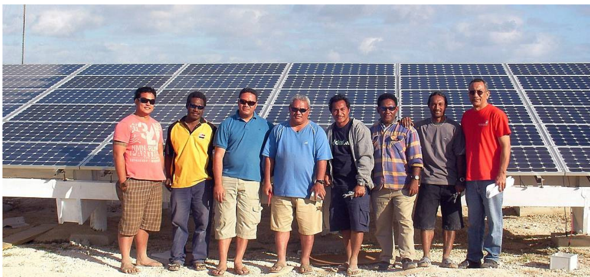
Some of the workshop participants at the hospital PV systems installation
